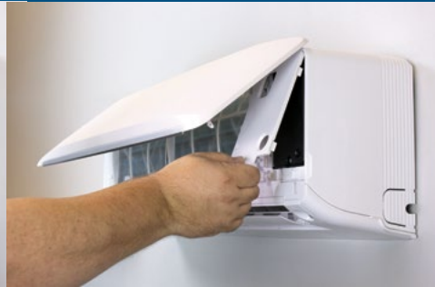
Remove electrical access panels (2)
