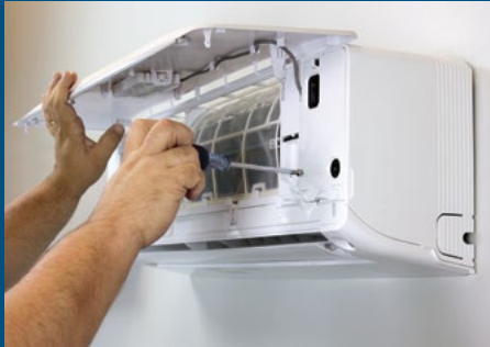
Back out electrical panel screws
