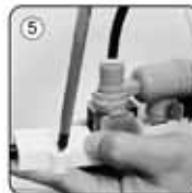
Close box and insert the screw into the protective box.
